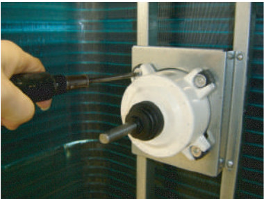
Remove the 4 mounting screws. Remove the FAN MOTOR.
